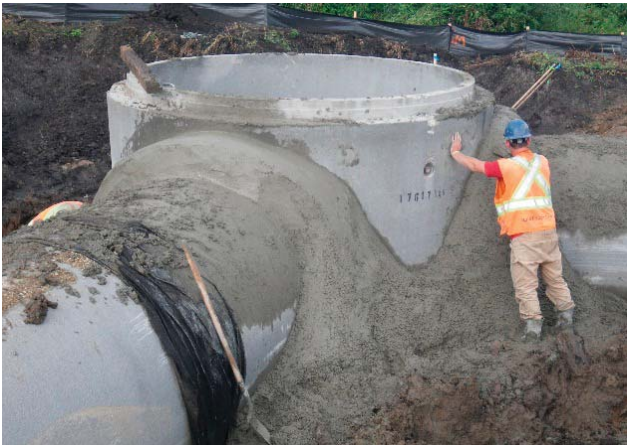
3 m diameter manhole being installed for the 1.5 m diameter storm sewer.
