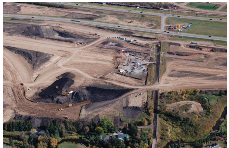
Worksite adjacent to QEII Hwy looking east
