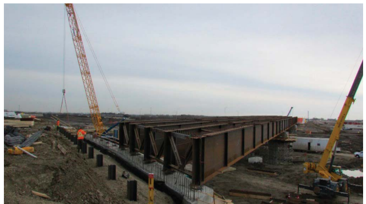
41 Ave SW over QEII Highway Bridge
