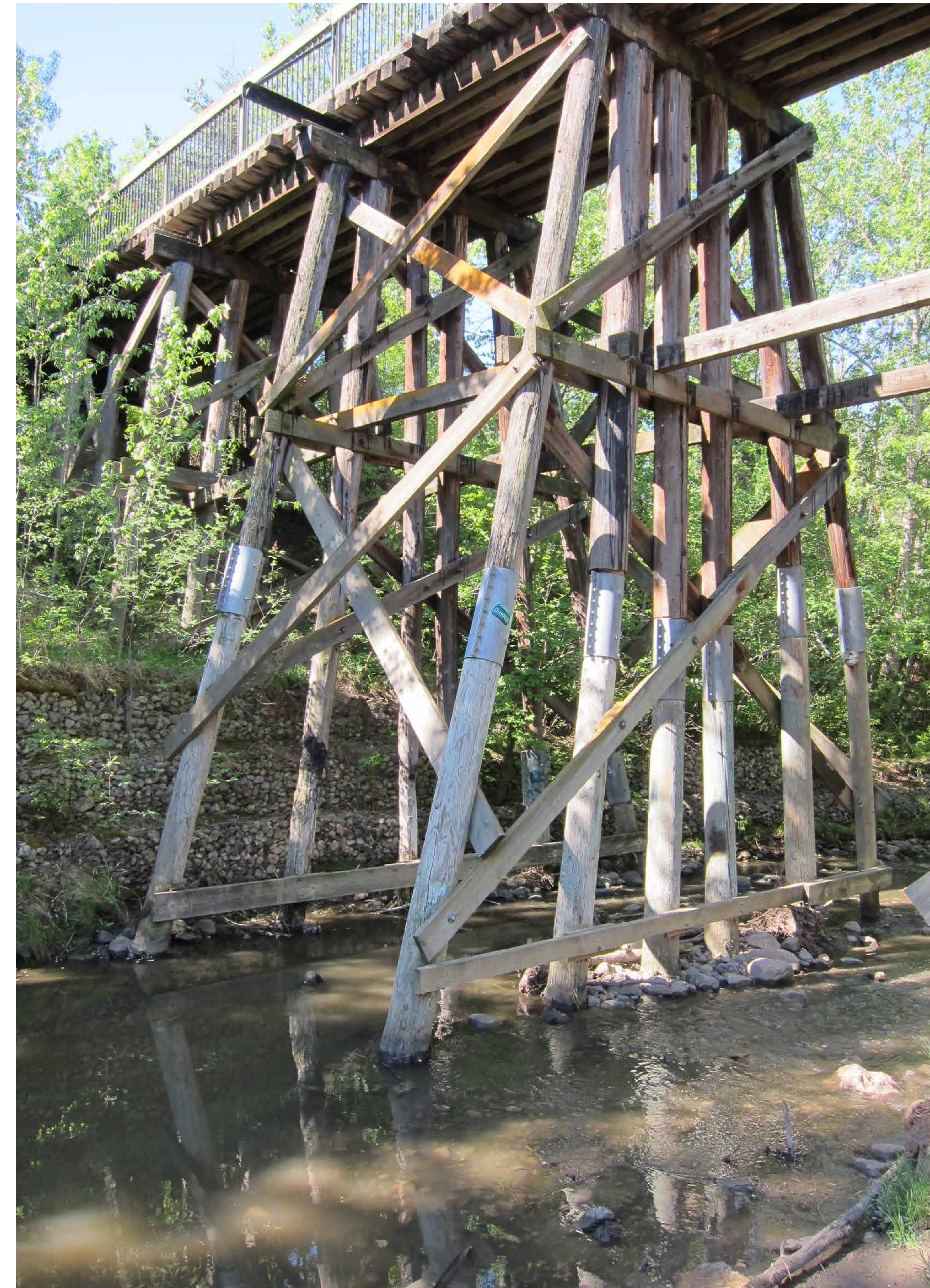
Bridge B033 - Piers in creek to be removed
