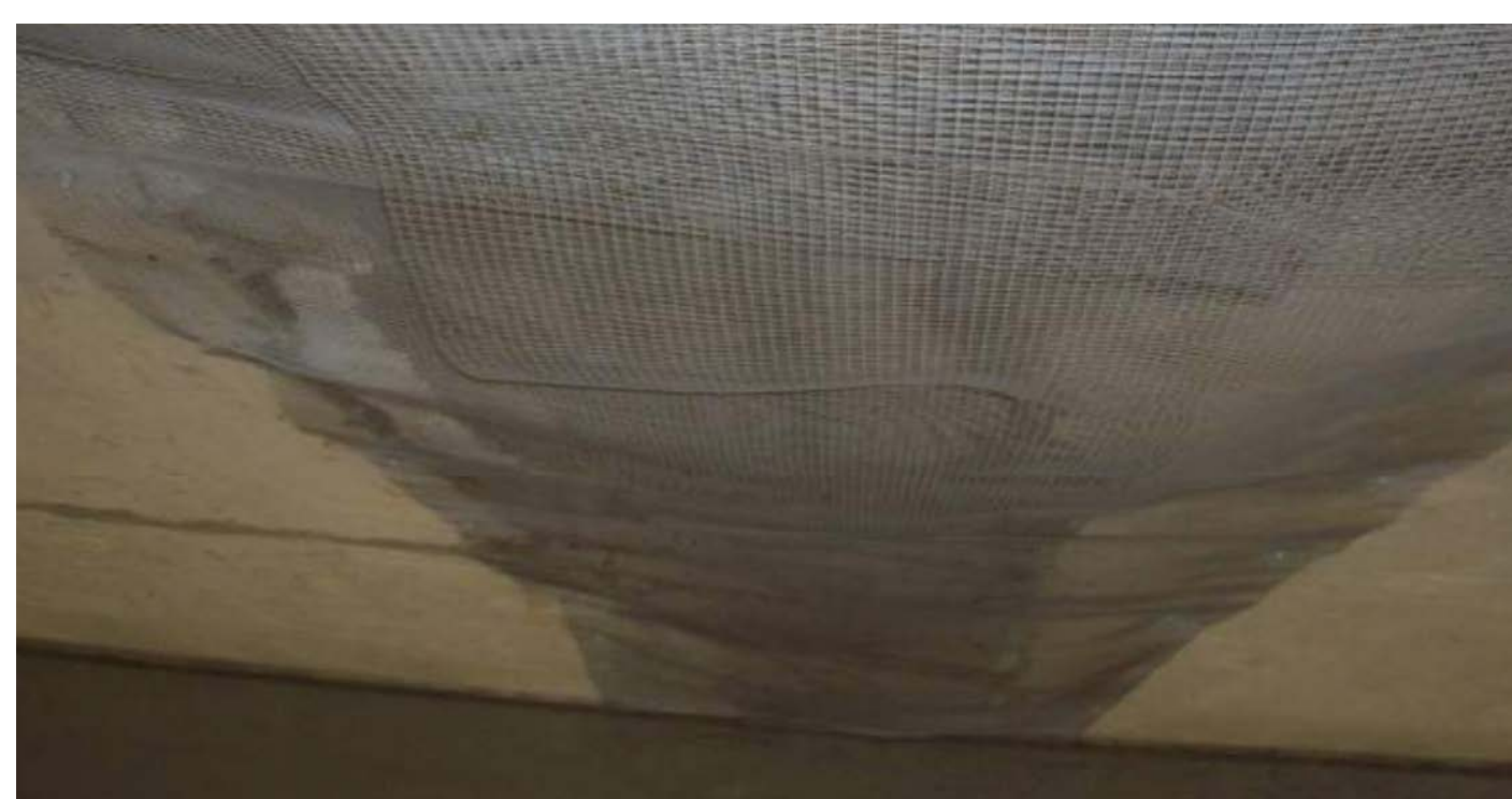
Concrete spalls at deck underside
