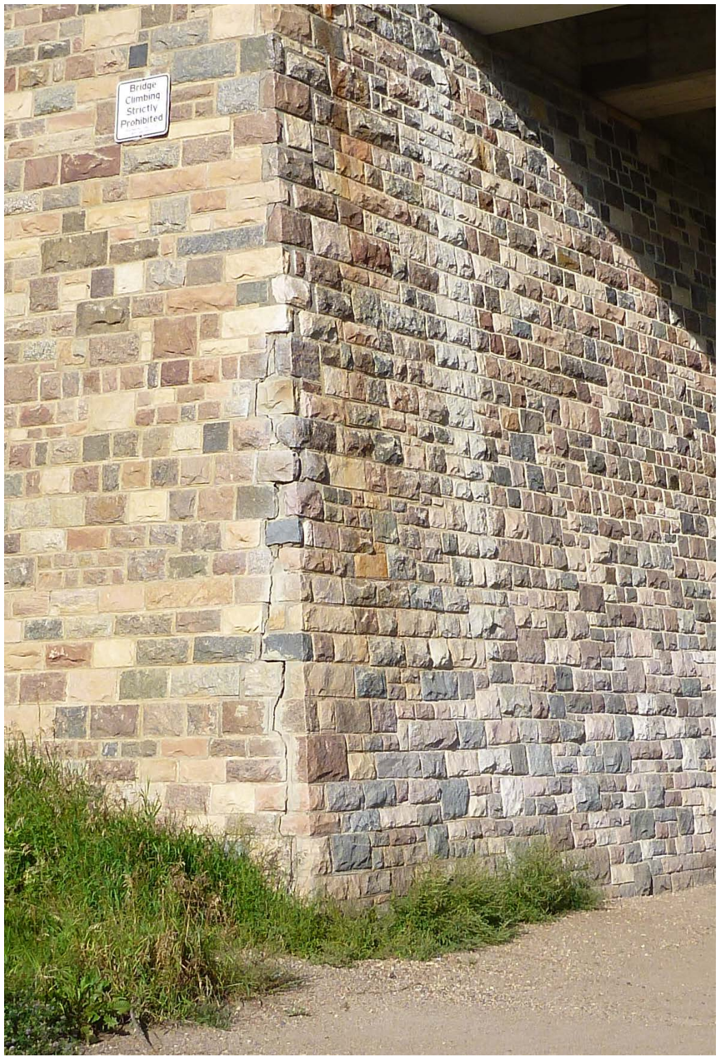
Stone wall separation at south abutment.
