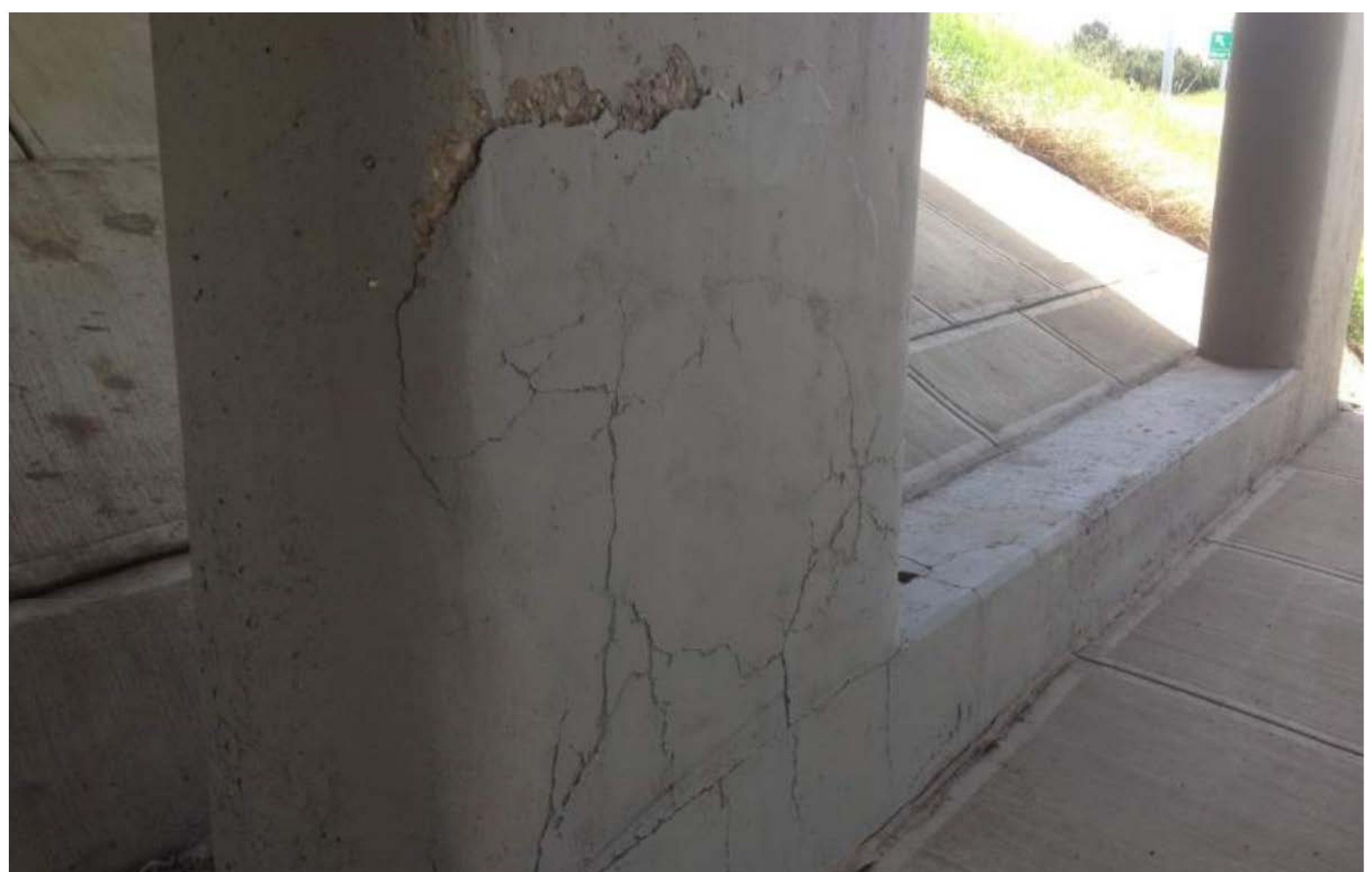
Cracking and delamination at pier
