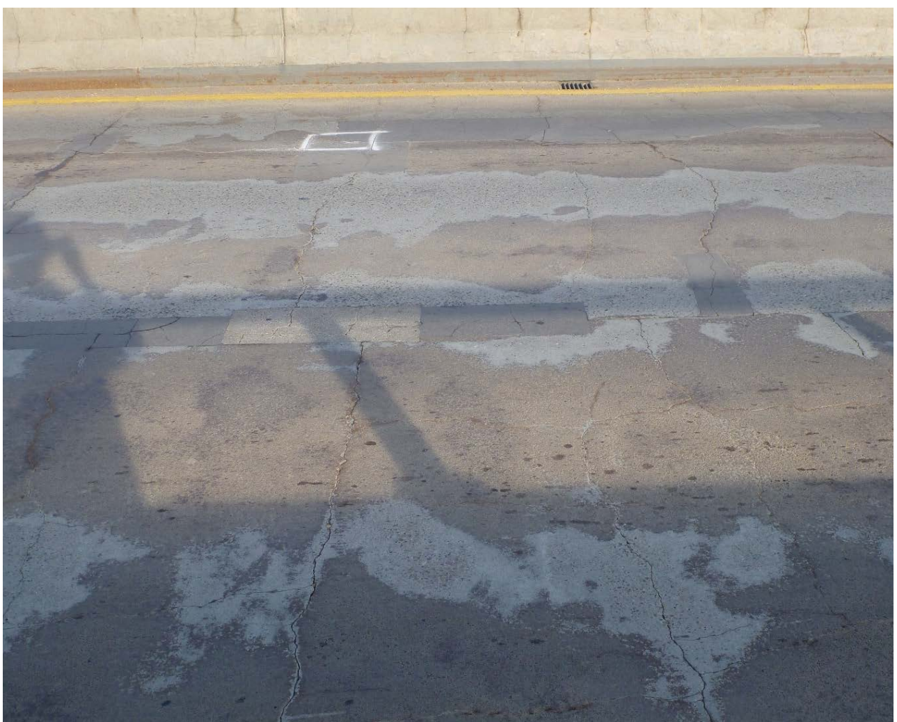
Significant deck cracking and spalling. Epoxy overlay is severely debonding.
