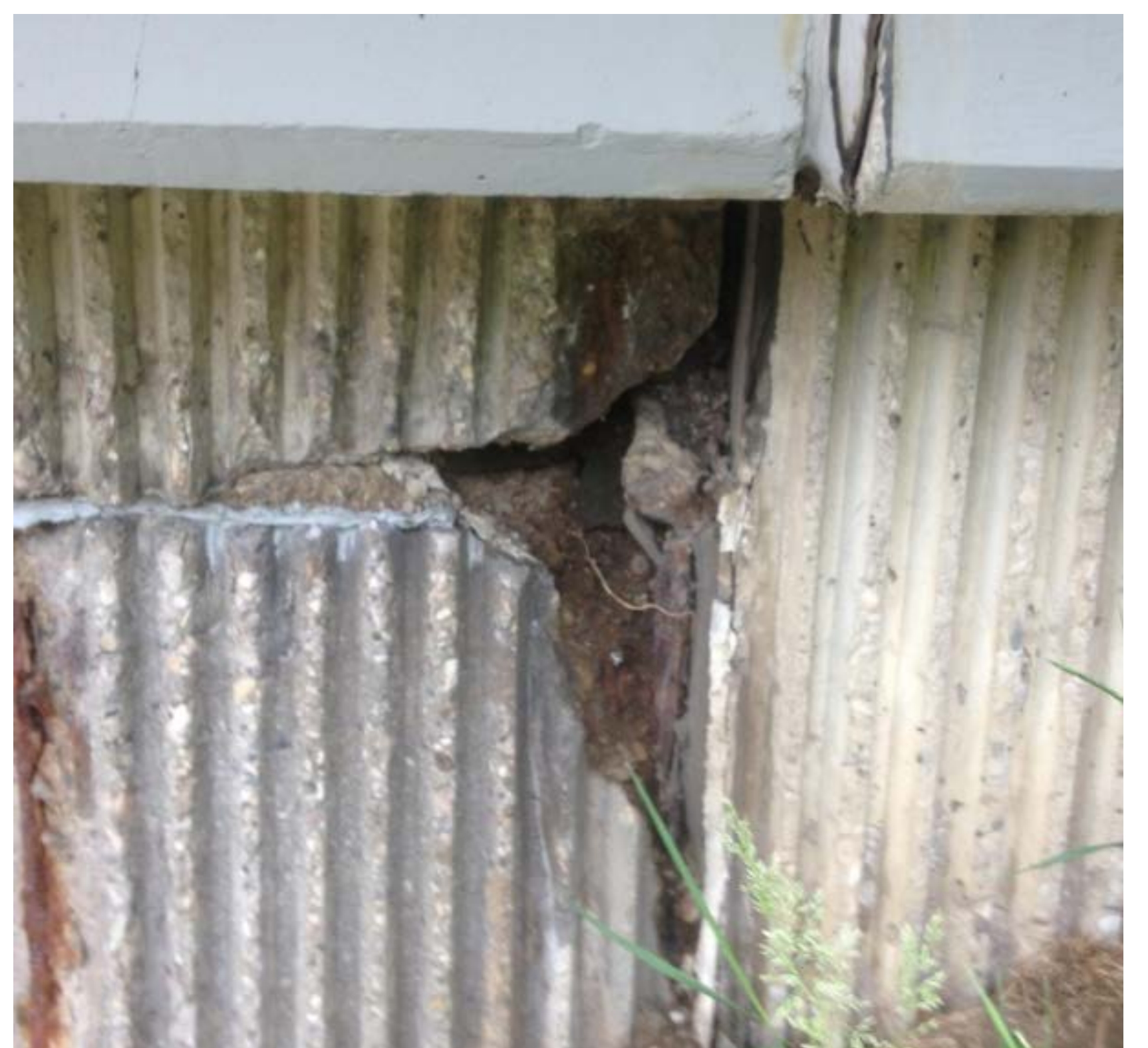
Deteriorated abutment concrete to be repaired
