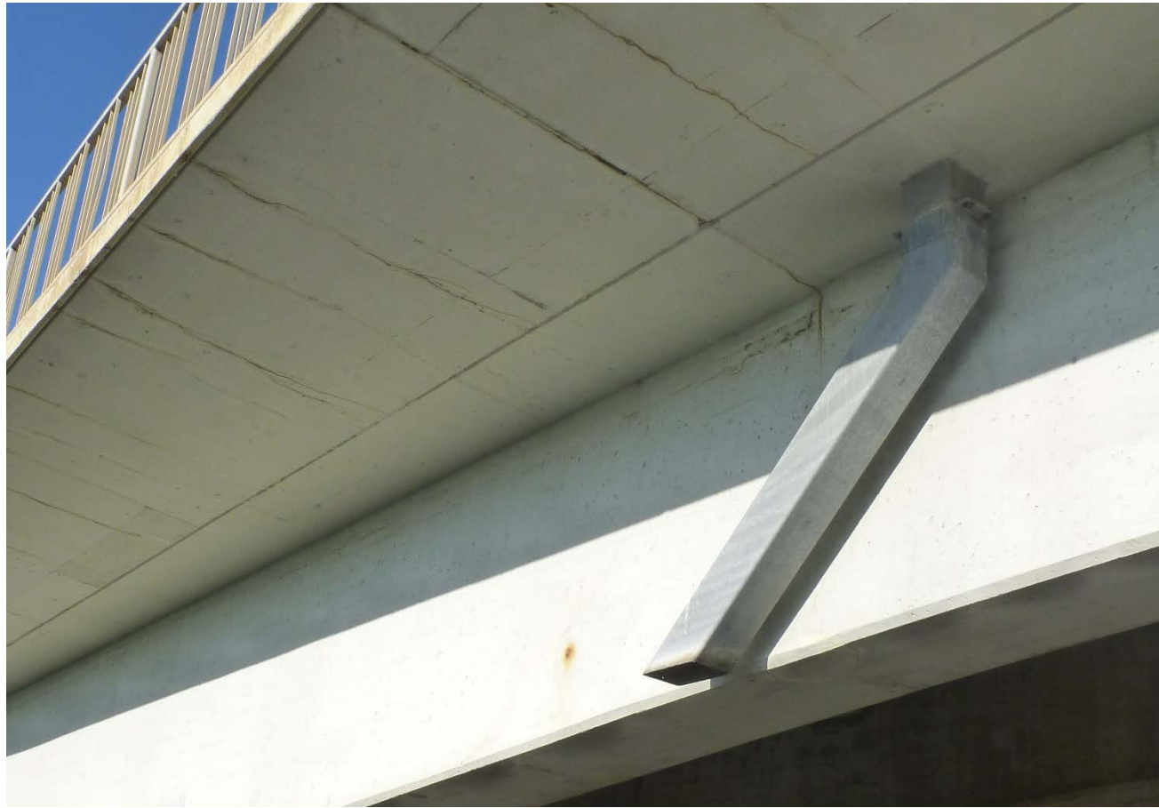
Cracking on underside of cantilever that supports sidewalks on east side of bridge. Cantilevers not post-tensioned.
