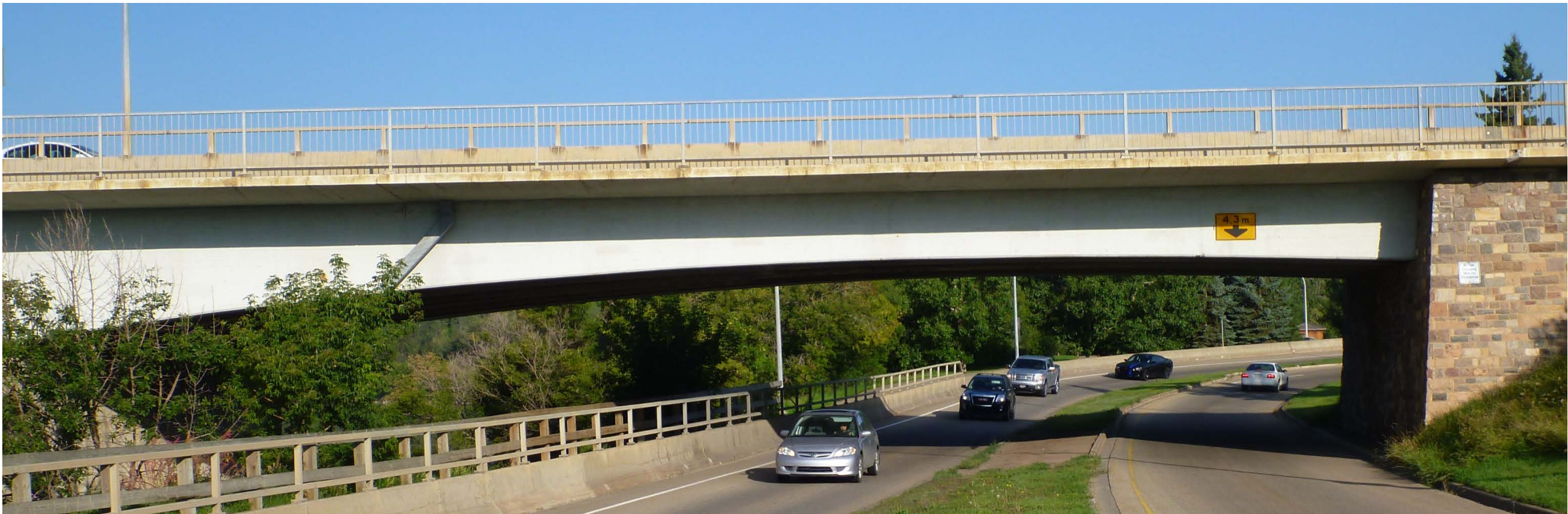
Girders are strength deficient and need strengthening or replacement for continual use.
