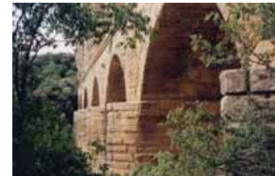
Le Pont du Gard, near Nimes, France from Roman times
