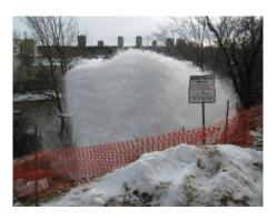
Water pressures in the water distribution system can range from 280 kPa to 1000 kPa. At an average pressure, a break on a 300mm water main can fill a 1m x 2m x 3m trench in 7 seconds. Thus, a water main failure can cause a lot of damage very quickly and pose significant risk to workers in excavations.
