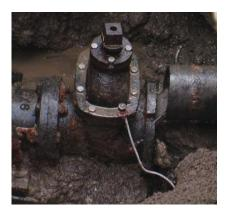
Joint failures can occur as the result of settlement or heaving, or excessive loading.
