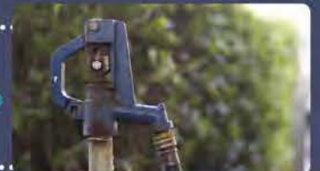
Dog Wash Station (can be a hydrant / hose bib with durable surfacing)
