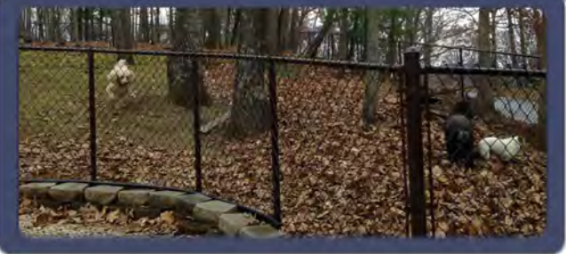
Chain link fencing with black vinyl coating
