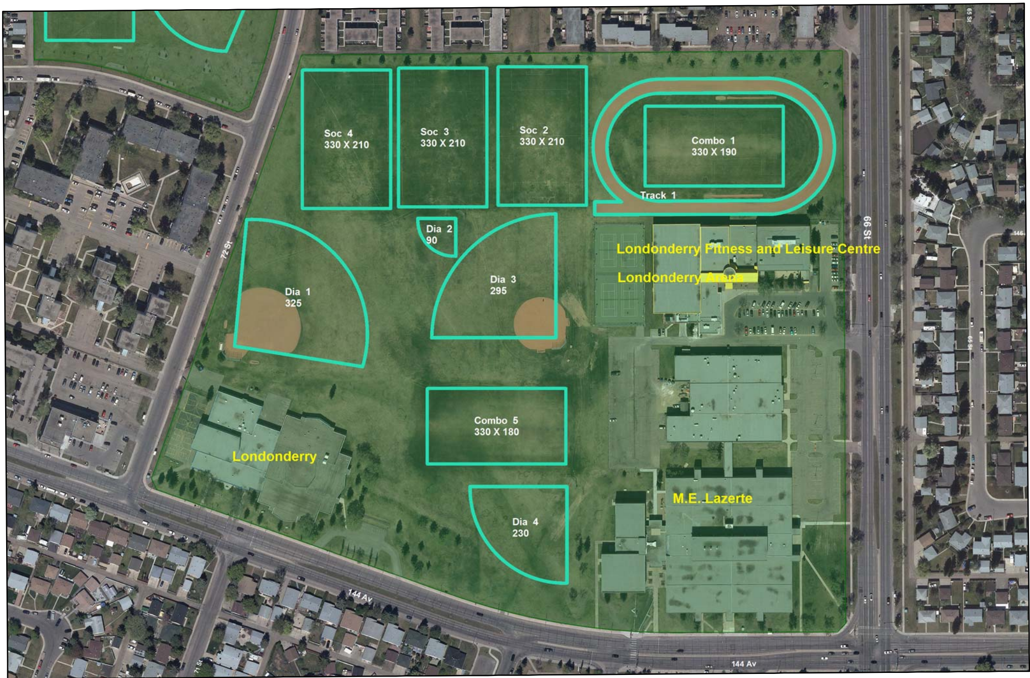
Londonderry / M.E. Lazerte Sports Fields 68 Street - 144 Avenue NORTHEAST
