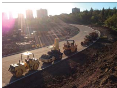
Paving of Queen Elizabeth Park Road
