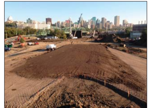
South side roadwork
