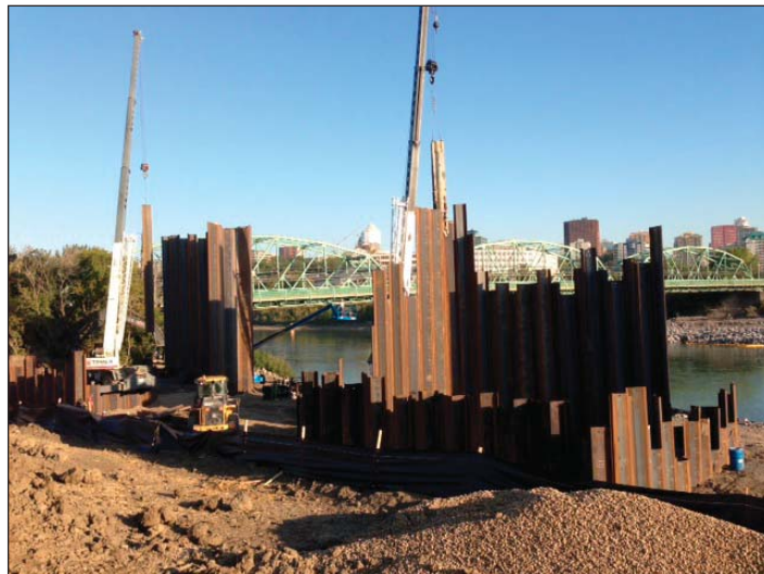
Sheet pilings on south side
