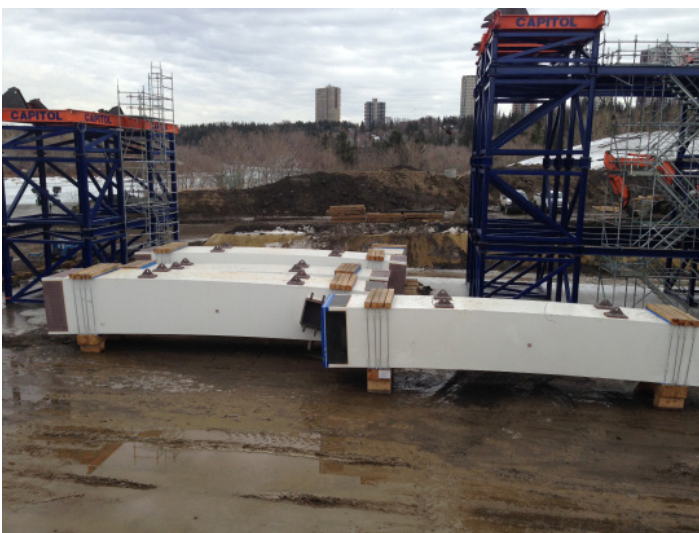
Central arch pieces in south side laydown area
