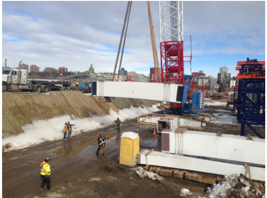
Central arch pieces are unloaded from trucks on the south side
