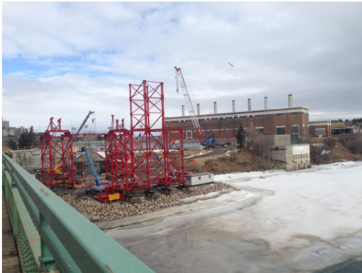
View of the north berm arch lift towers from the old bridge
