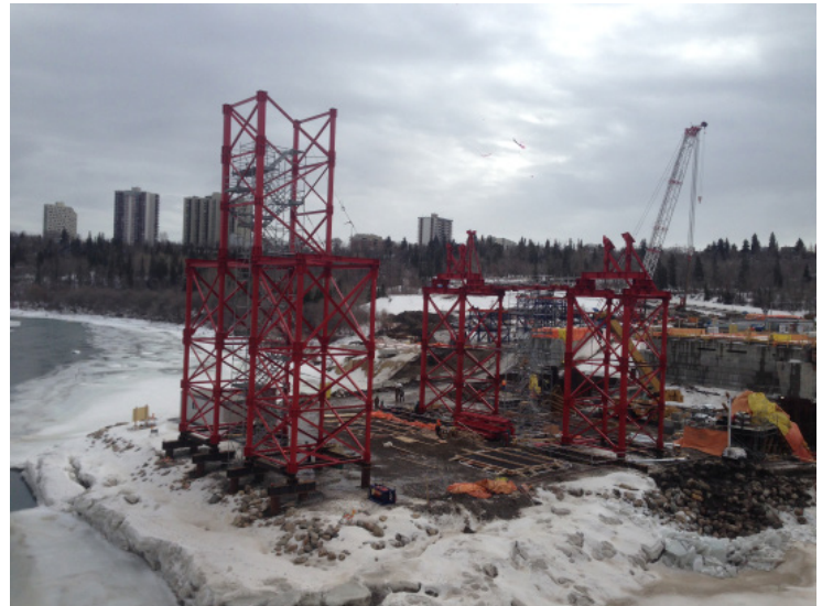
Arch lift towers on the south berm
