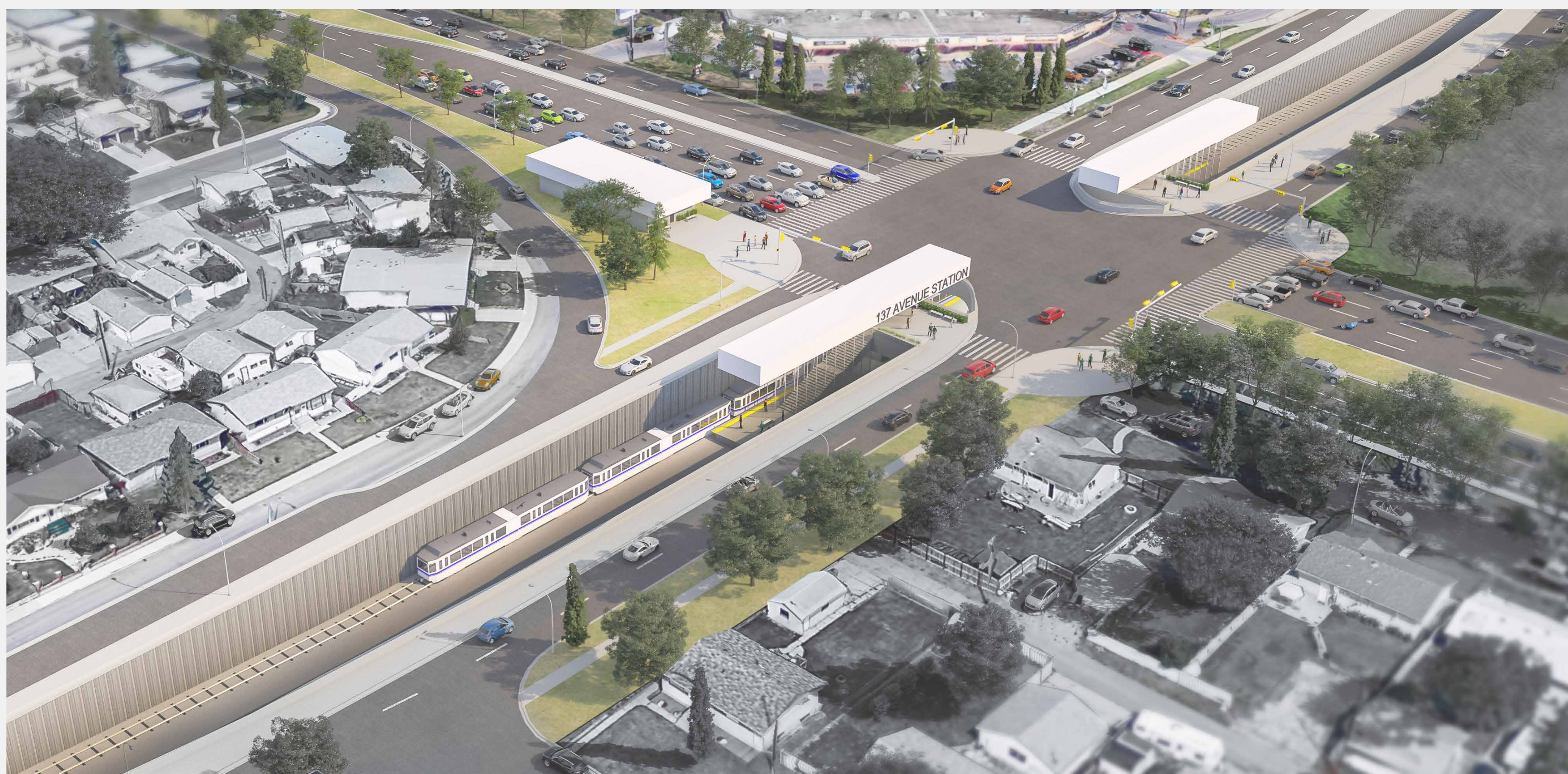
the 137 Avenue trenched option shown above provides an example of how a similar trenched option at 127 Street and 153 Avenue might look
