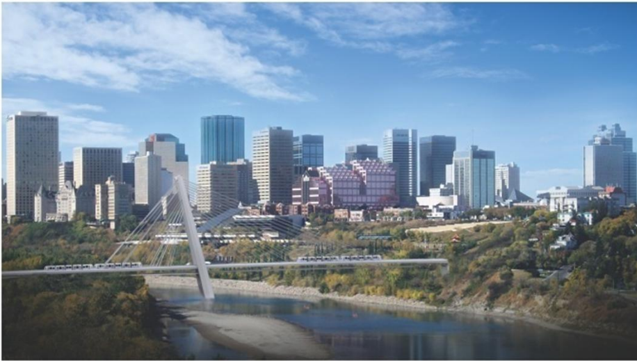
Option 1 - Cable stayed bridge looking Northwest
