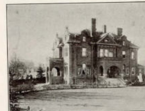
J. A. McDougall's House, Victoria and Third St. EB-26-223
