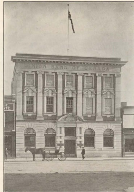
UNION BANK OF CANADA, JASPER AVE. EAST
