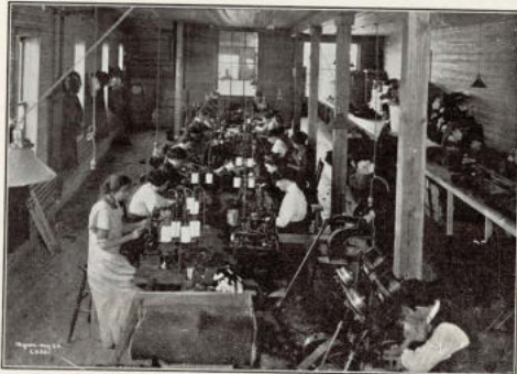
INTERIOR OF FACTORY AT 328 NAMAYO AVE. EB-26-271
