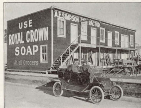
A. E. SIMPSON'S SHOP AND YARD, 739 SECOND ST. EB-26-272
