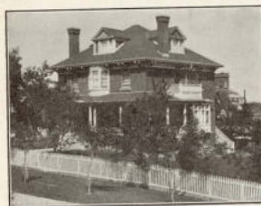
Government House, Third Street EB-26-347
