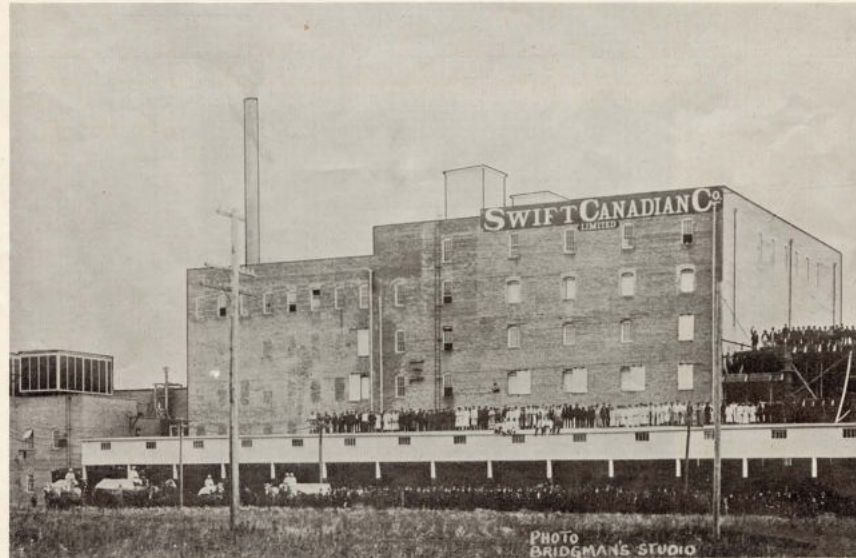
Swift Canadian Co.'s Parking Plant, Employing 330 People
