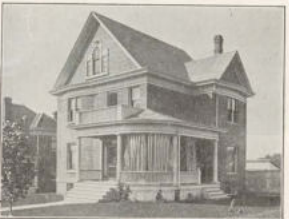
J. I. Mills House, Sixth Street EB-26-361
