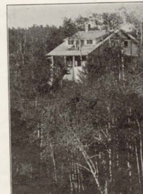
House in Wadleigh Park (Groat Estate) EB-26-346
