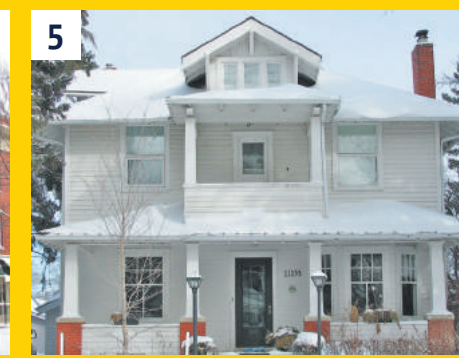
5 11153 – 64 Street (1912) Residence of Ernest William Morehouse, architect for Magrath-Holgate & Co. Ltd. Morehouse designed many Highlands homes, including the Magrath and Holgate residences, and the Gibbard Block.
