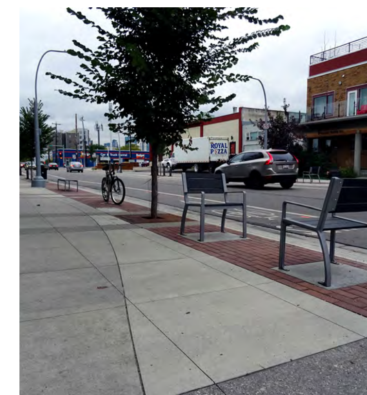
2016, 116 to 119 Street Construction
