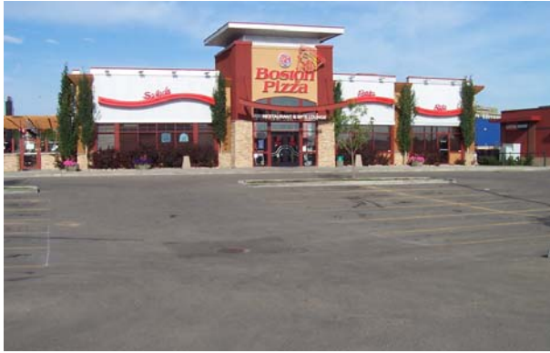
Asphalt repair around the catch basin
