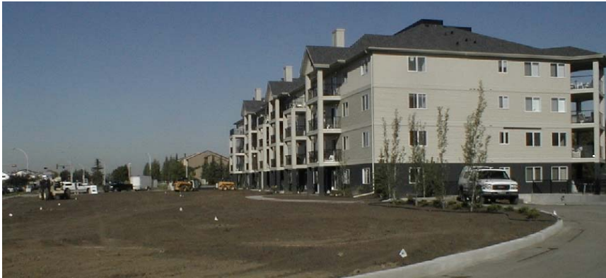
Final Grading in progress at a condominium / multi-family site
