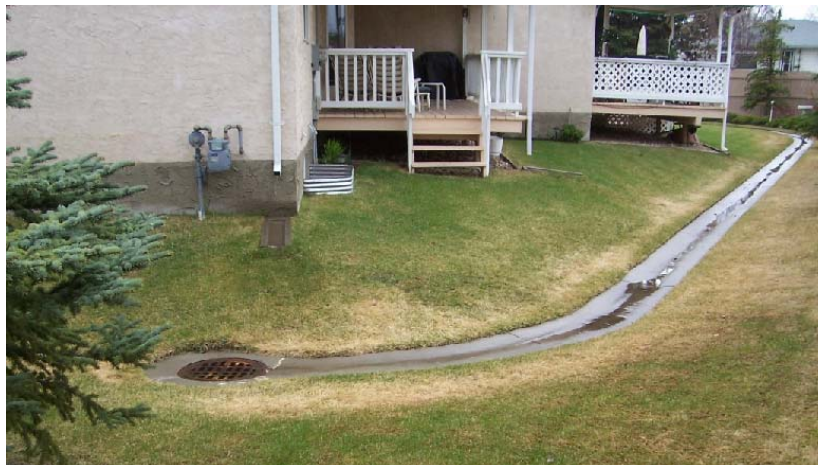
Condominium site with a concrete drainage swale that drains into a catch basin
