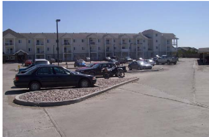
Example of concrete grading on a condominium parking lot
