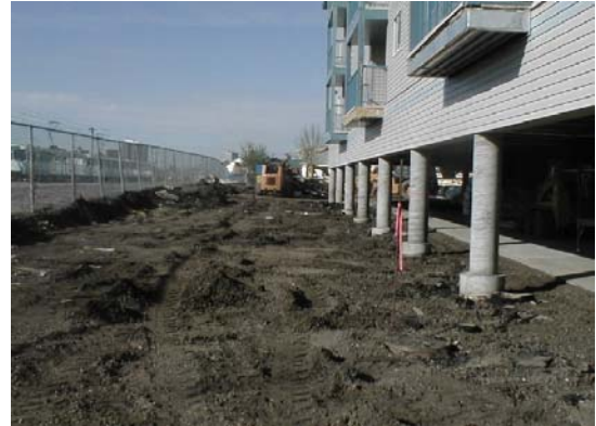
Grading in progress at an apartment / multi-family project
