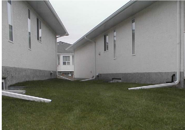
Downspouts with extensions at condominium
