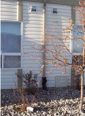
Downspout at an apartment connected to storm service
