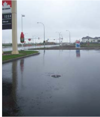
Drainage into a catch basin during a storm
