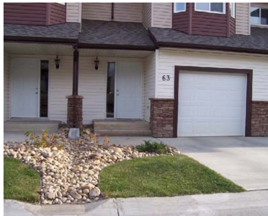
Grading away from the wall on a row housing project
