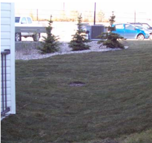
Grass swale into a catch basin at an apartment site
