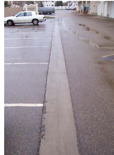
A concrete swale within a parking lot
