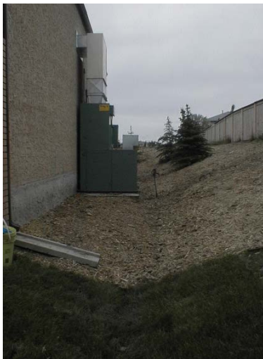
Internal drainage swale in between the building and property line at a commercial site
