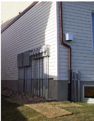
Positive slope away from building
