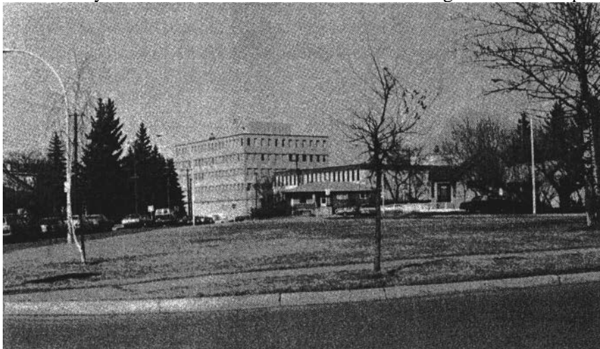
Open space at Wadhurst Road looking north.
