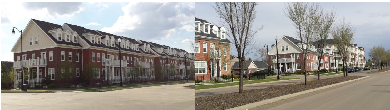
Photos: Griesbach Row Housing, Griesbach
