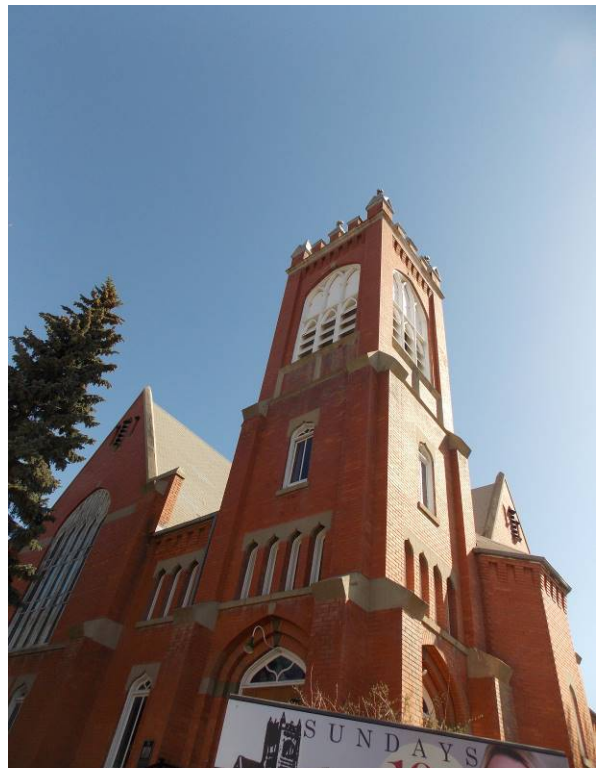
Ensuring the preservation of existing historic
