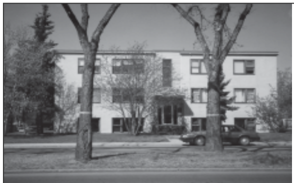
Typical older apartment
