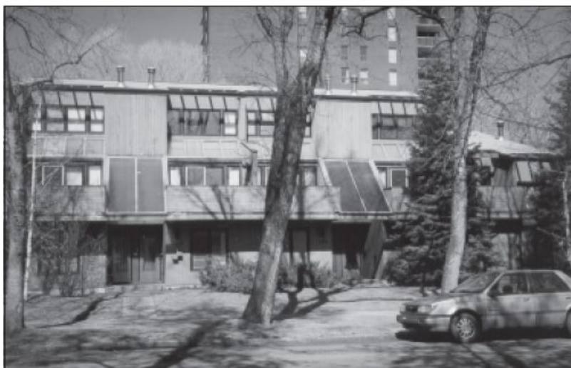
Apartment housing uses regular front entrances and setbacks and features to create interest on the street
