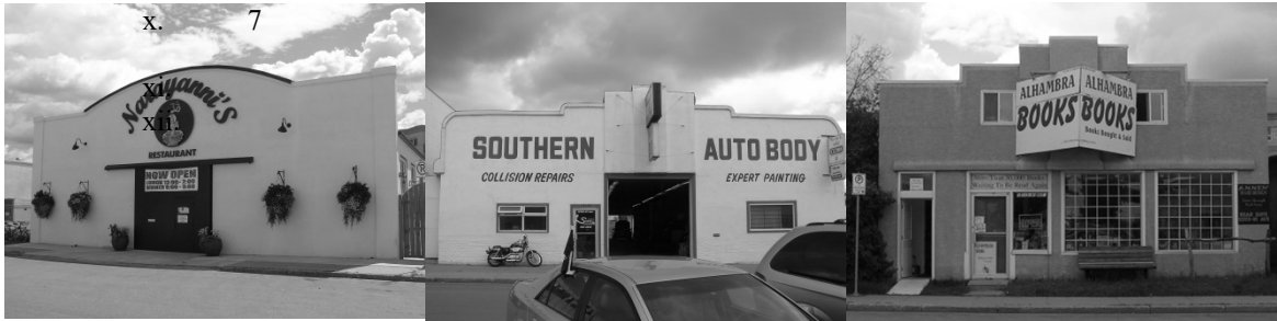
Figure B. False Façades in West Ritchie
