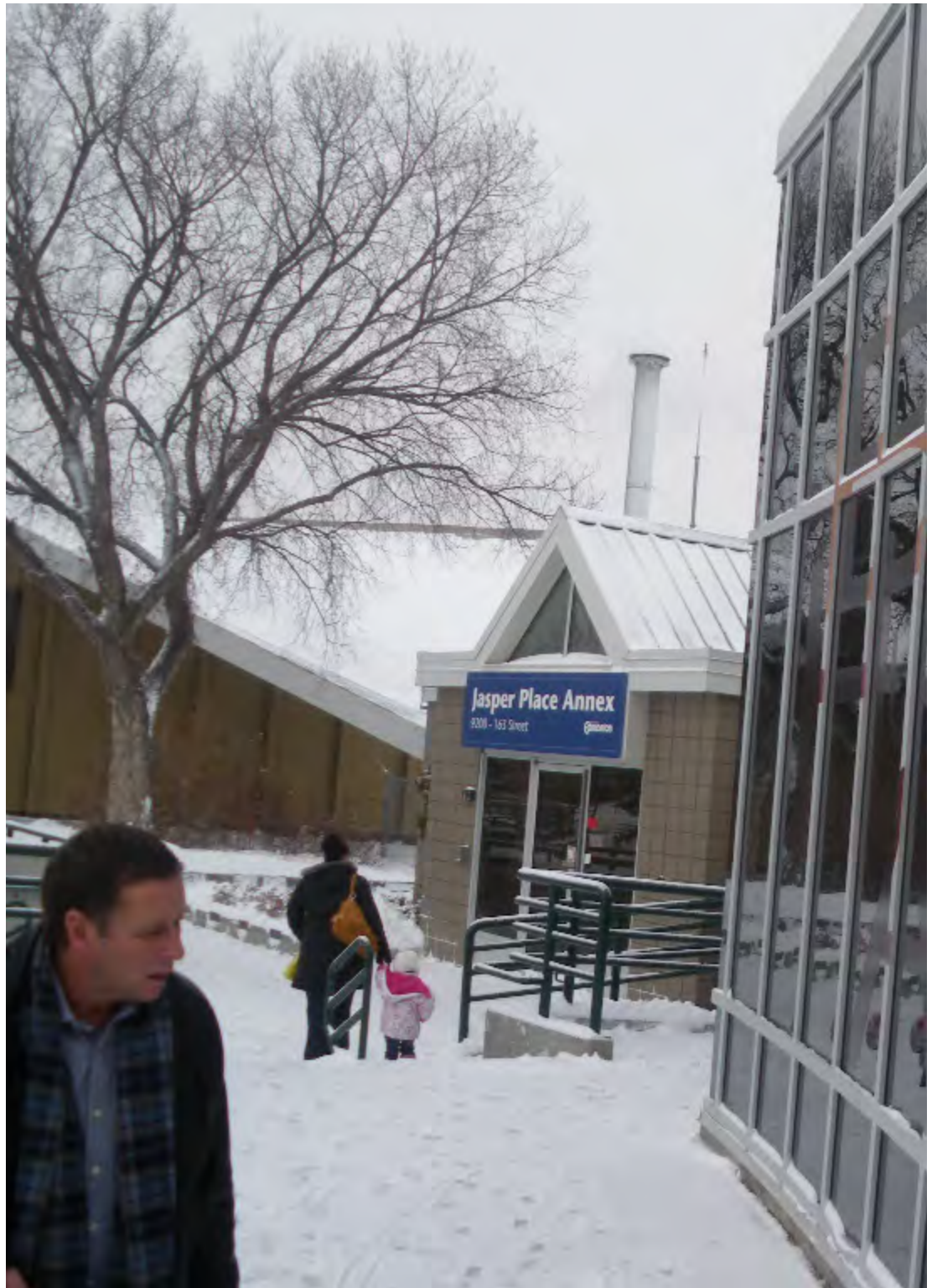
Composite exterior view of the existing Jasper Place Fitness and Leisure Centre, Jasper Place Annex and the Bill Hunter Arena.
