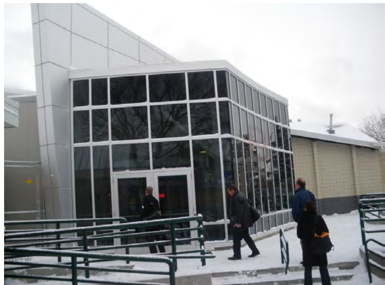
Below: Exterior view of the new entrance to the Bill Hunter Arena
