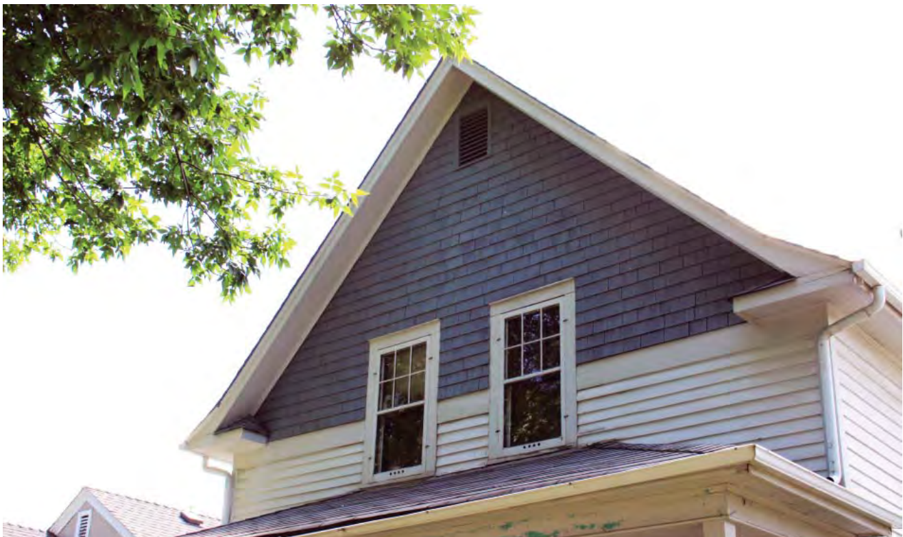
>> Front view of second storey
