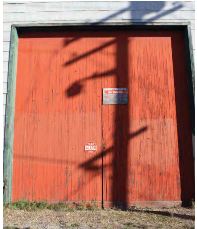
>> Doors on west elevation
