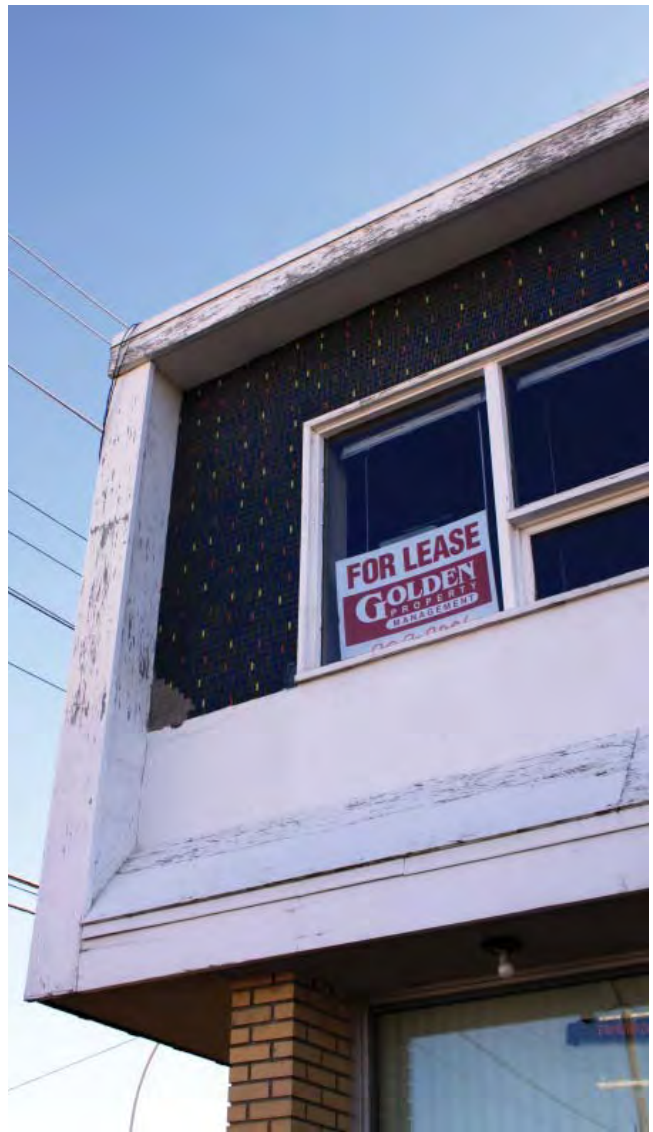
>> Second storey window and tile
