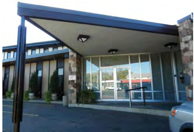
>> View of entrance from north
