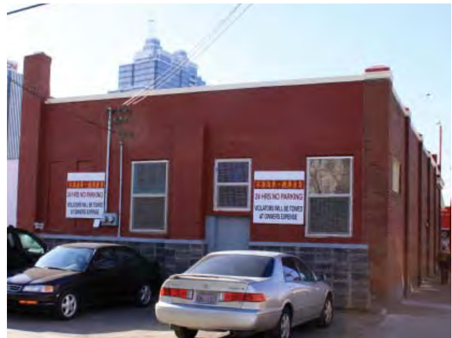
>> Rear of building
