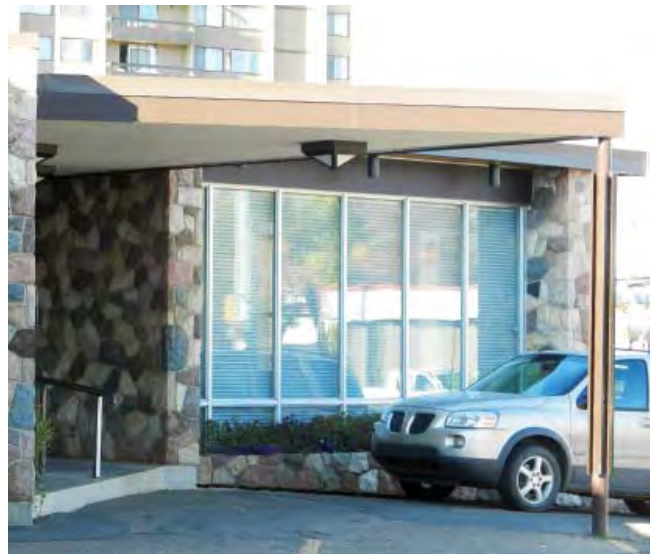
>> View of entrance from east
