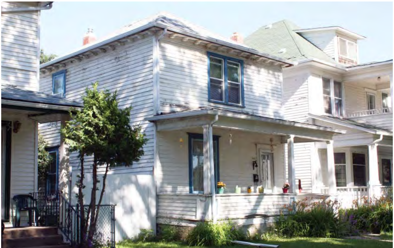
>> South and east elevations
