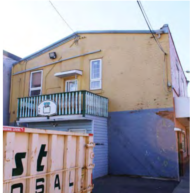
>> Rear of building facing east
