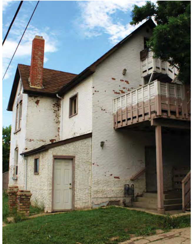
>> Rear view from northwest
