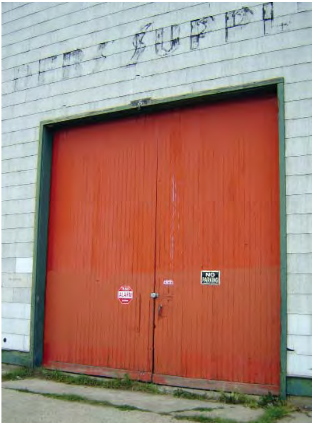
>> Doors on east elevation
