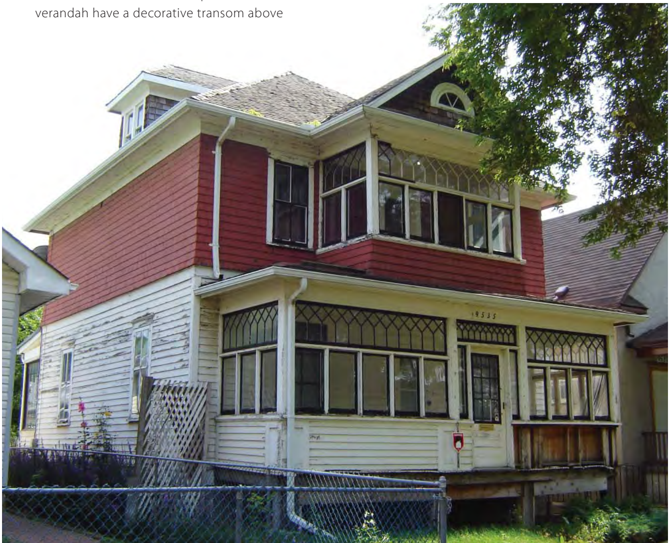
>> North and east facades
