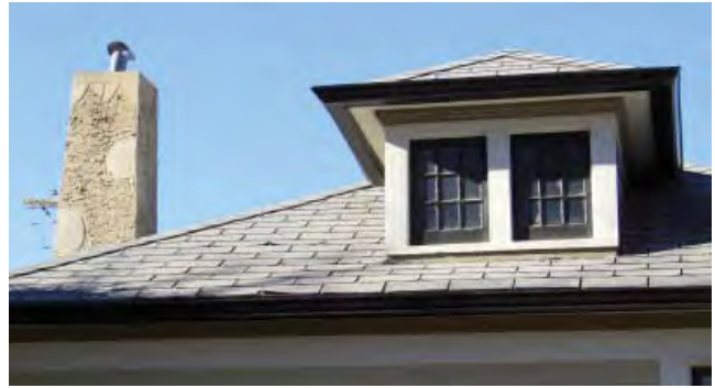
>> Chimney and dormer
