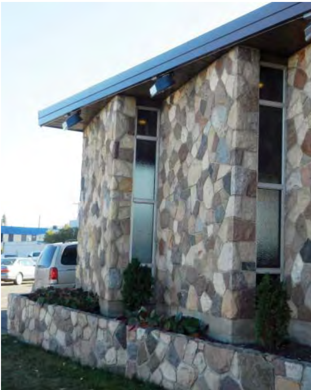
>> Staggered wall along 111 Avenue
