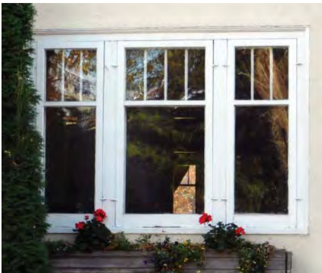
>> Three-panel window on façade
