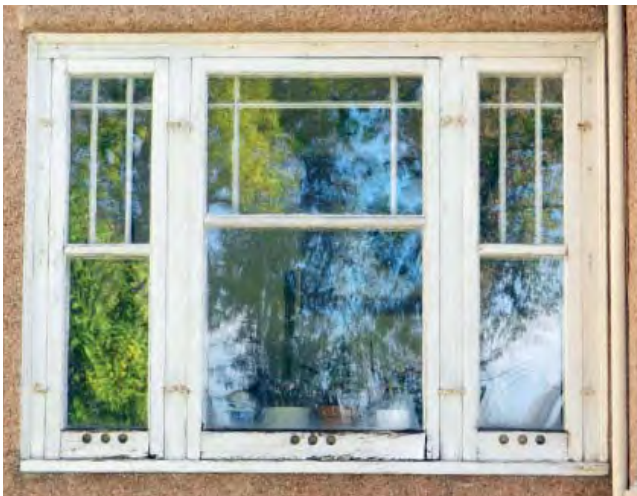
>> Front window north of entry
