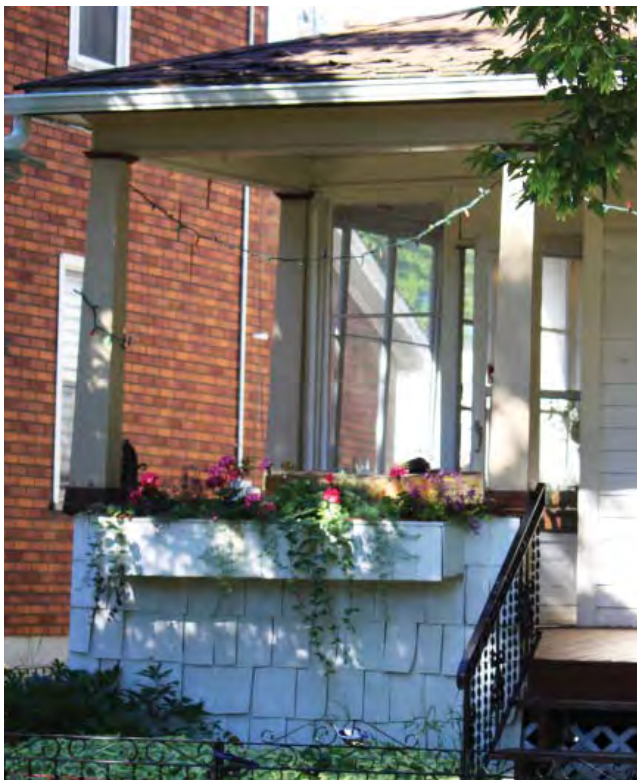
>> South end of verandah
