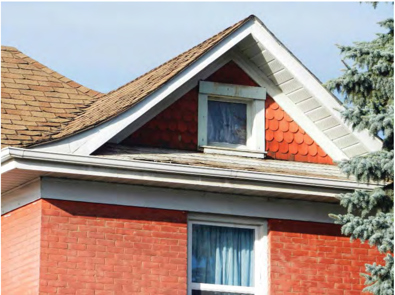
>> Roof line and gable window
