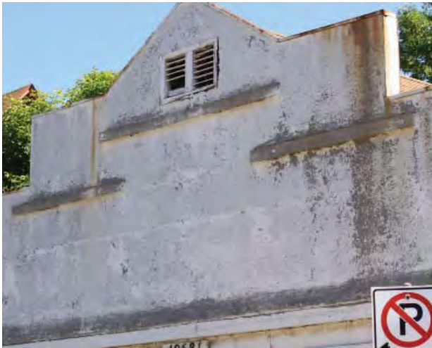
>> Boomtown façade detail
