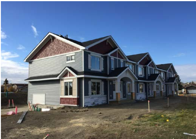
Bears paw site under construction
