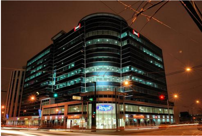
Figure 11: Intact Insurance Building, 10830 Jasper Avenue
