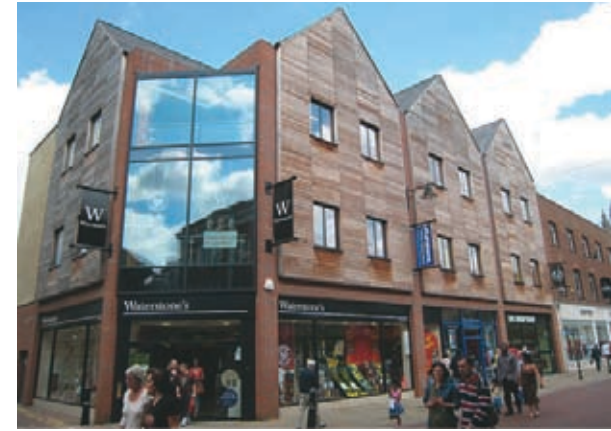
New developments are encouraged to use honest materials and creative parameters, as well as incorporate art into façades.
