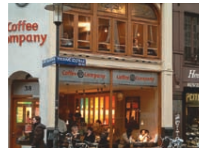
Use specific design options to restore or rehabilitate existing buildings
